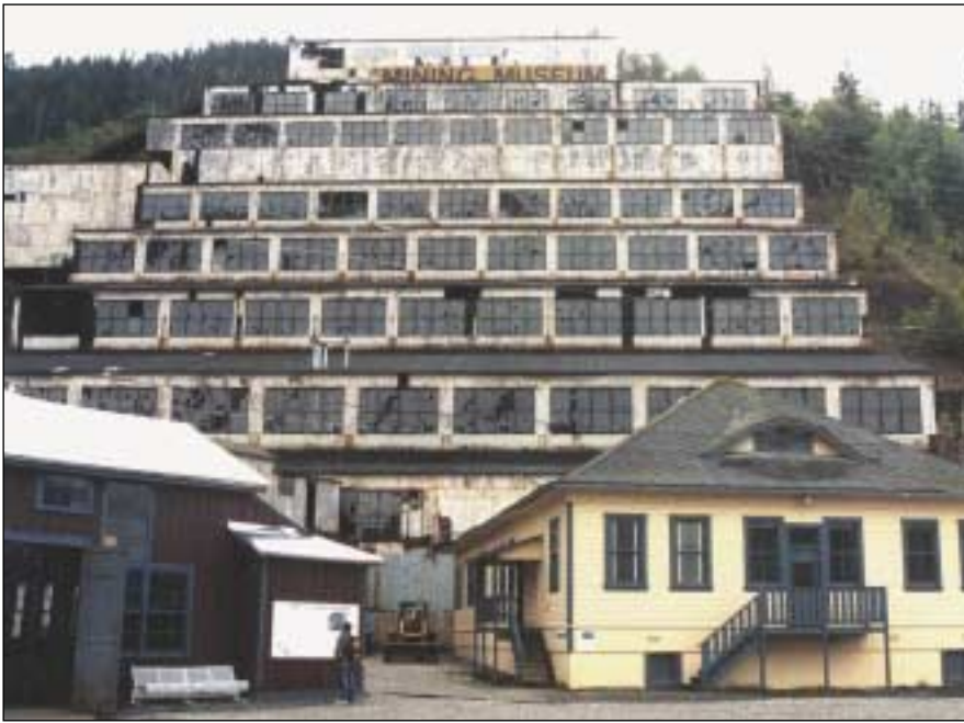
Bottom left and above: the Britannia mine, about 10 km south of Squamish on Hwy 99, was the largest copper producer in the British Commonwealth. Left: View of Howe Sound from the mine. Acid mine drainage continues to discharge into Howe Sound to this day. Remediation plans include treatment of the acidified mine water and contaminated soil, and revegetation and stabilization of the hillsides. The Britannia mine was designated a national historical site in 1988. Today, the site operates as a mining museum and tourist attraction.
